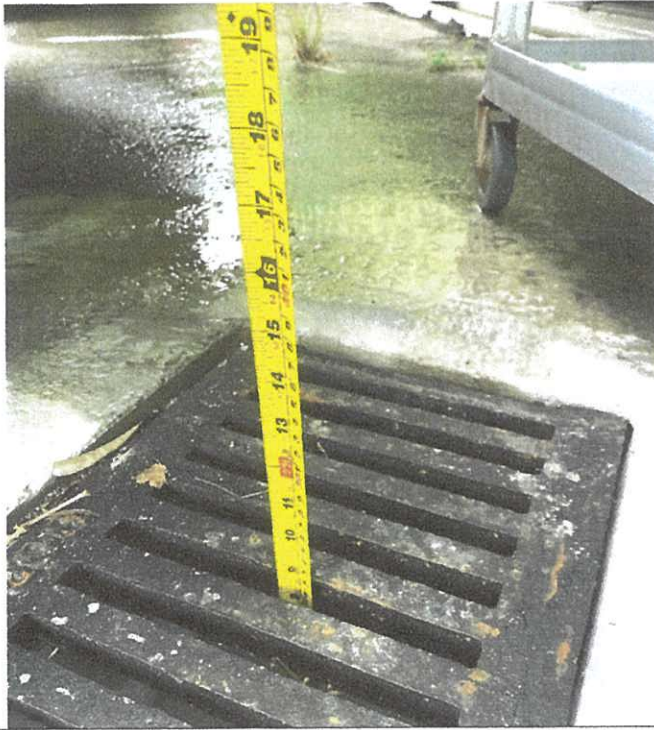
P3: shows the depth of channel at start (225mm)
