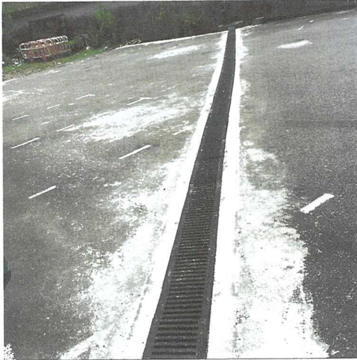
P1: shows overall view of the drainage improvement at car park
