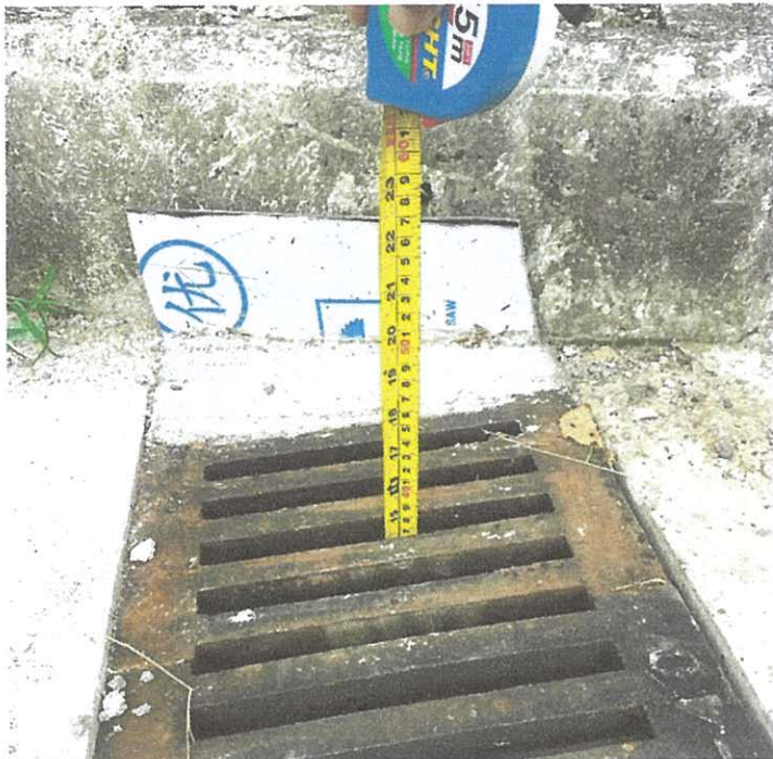
P4: Shows the depth of channel at near the manhole ((375mm)
